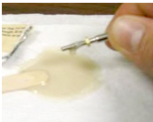
Figure 2.7-5: Putting Epoxy Onto the Nut and Threads of the Shaft Coupler
